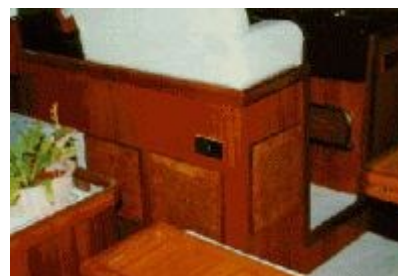
The pictures show the use of the air distribution grills, their shape and some of the possible installations. As the cold air is heavier than warm air, the cold air falls therefore the cooled air should be dispersed across the deck head or at least upwards. This is achievable also by realigning the grill blades. The air grill has also a high impact on the inside decor.
