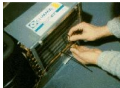
Picture 17: The bulb is installed on its support in the air intake section of the air-conditioner.
