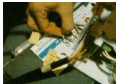
Picture 21: Mains cable and pump cable must be connected to the electrical box. Make sure that each wires goes into its terminal and that the fixing screw block the copper wire correctly.
