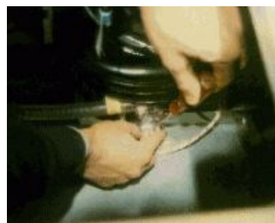
Picture 18: The air-conditioner is installed in its space and fastened by means of four practical brackets in stainless steel.
