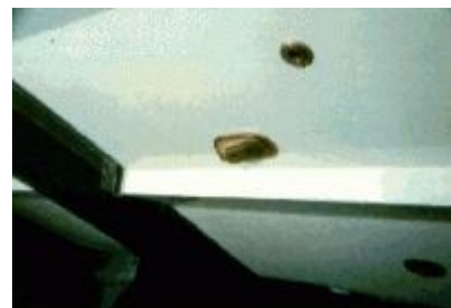
Picture 10: The through hull intake installed in the aft section. The scoop type intake oriented forward helps the flow and will clear the sea water circuit of air if it gets into the circuit. If installed facing aft it will prevent a proper functioning of the pump as the circuit will be emptied while cruising.
