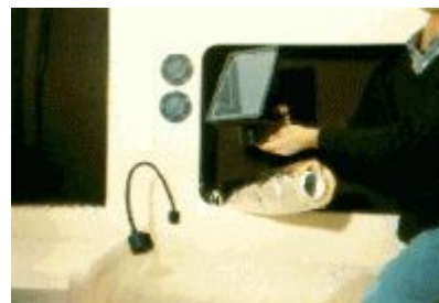
Picture 5: As explained in the text, round closable grills are simply installed by making a hole in the wall. On the opposite side of the wall it is installed a distribution plenum connected to the air duct.
