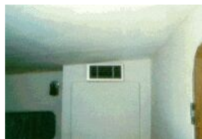
Picture 6: The air is ducted, through a connecting plenum to the owner's cabin and to the dinette; the grill for the owner's cabin is just above the locker door. You must remember that cold air falls and must be delivered at high level.
