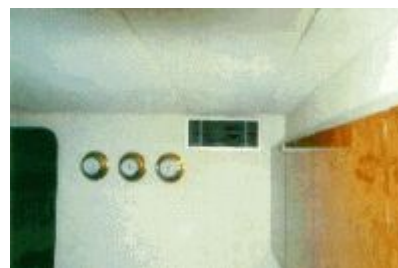
Picture 7: Above figure shows the delivery grill for the dinette, installed in the forward bulkhead; especially for the "day area" zones it is
