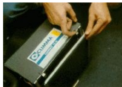
Picture 16: The air filter taken out from its plastic bag is installed in the front of the air-conditioner after the thermostat bulb has been fixed on its support. The thermostat senses the ambient temperature more effectively if its sensing bulb is installed in the return air.
