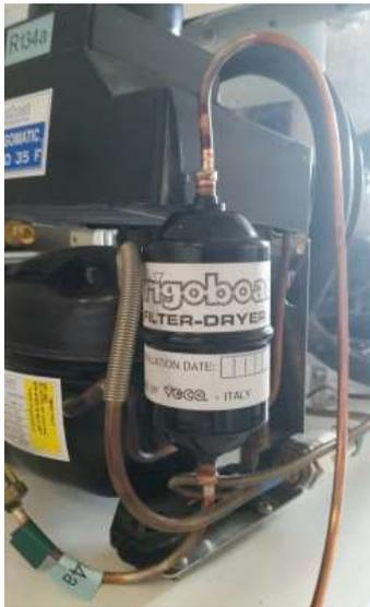
The filter drier works correctly in the vertical position with the arrow indicating direction of flow as shown in the enclosed photo. Filter drier should be secured with copper pipe not chafing or vibrating.
